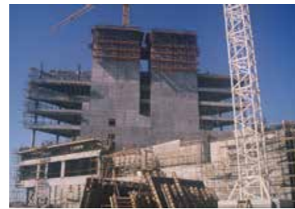
Dubai Chamber building under construction.
